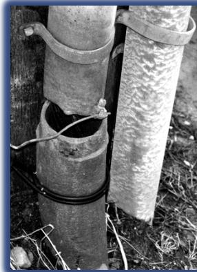
Steel U-Guard required grounding, strapping, and does not have belled ends.
